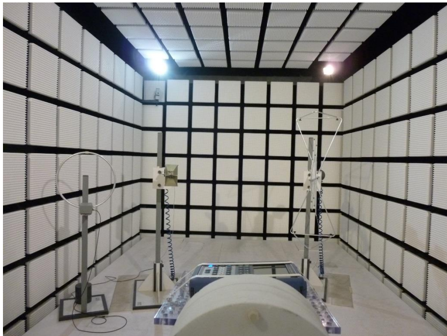
Photo 7: Fully anechoic chamber
