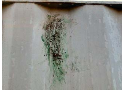
Figure 2-4 Dirty, greasy mount location
