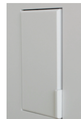
Correct: Dimmer/switch protrudes from faceplate.
