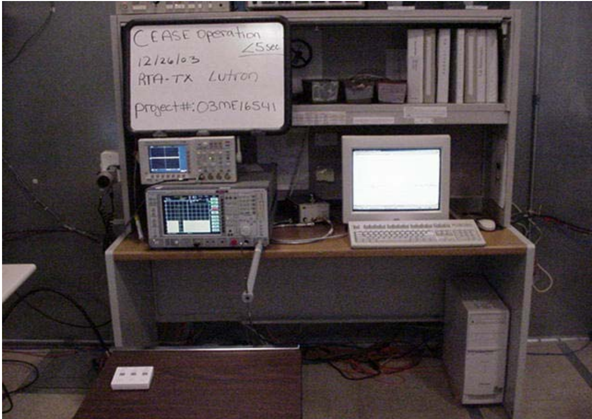
Cease Operation in < 5 Seconds Test Set- Up
