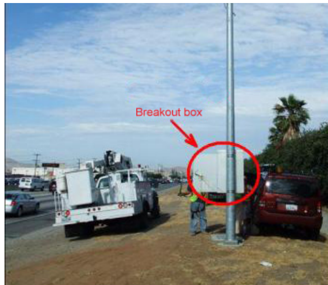
Figure B-1: Typical Installation
