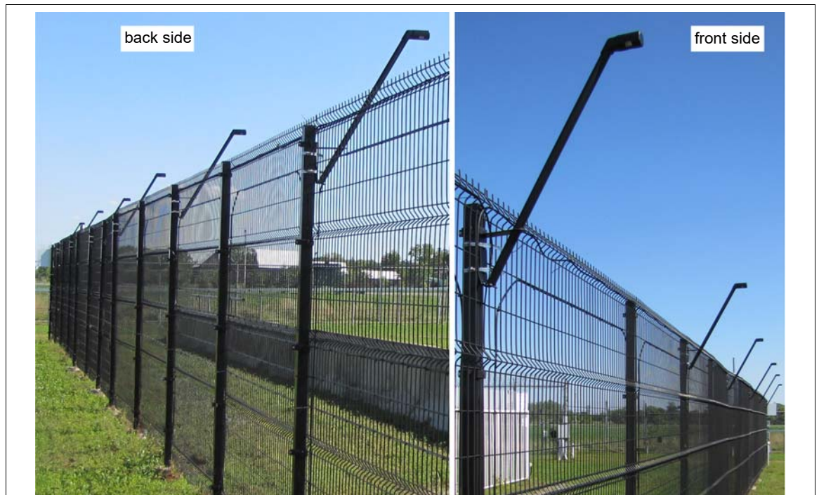
Figure 16: Welded-mesh fence with luminaires
