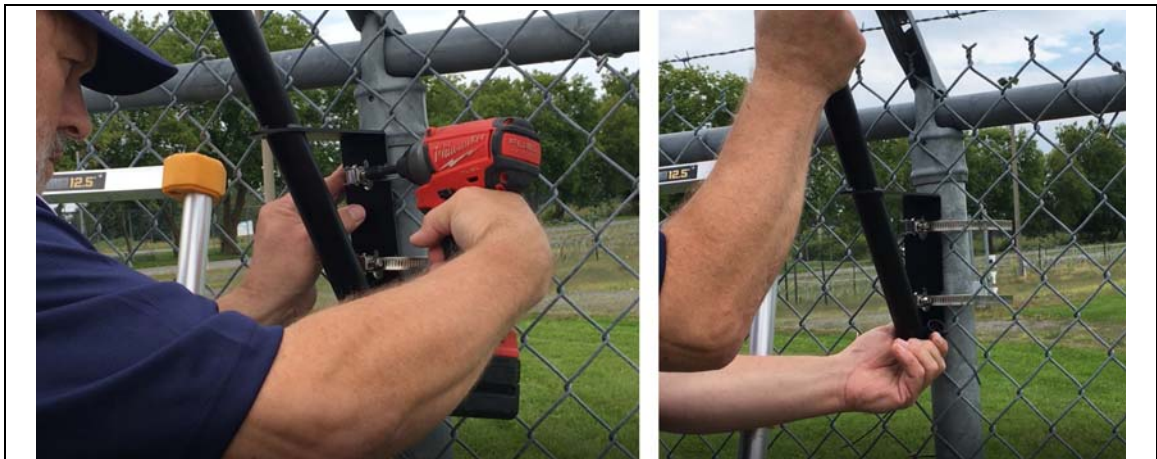
Figure 11: Luminaire installation steps 3 & 4
