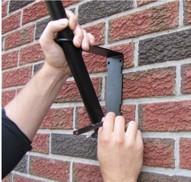
Figure 19: Surface mounting luminaires
