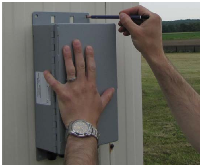
Figure 32: Surface-mounting the enclosure
