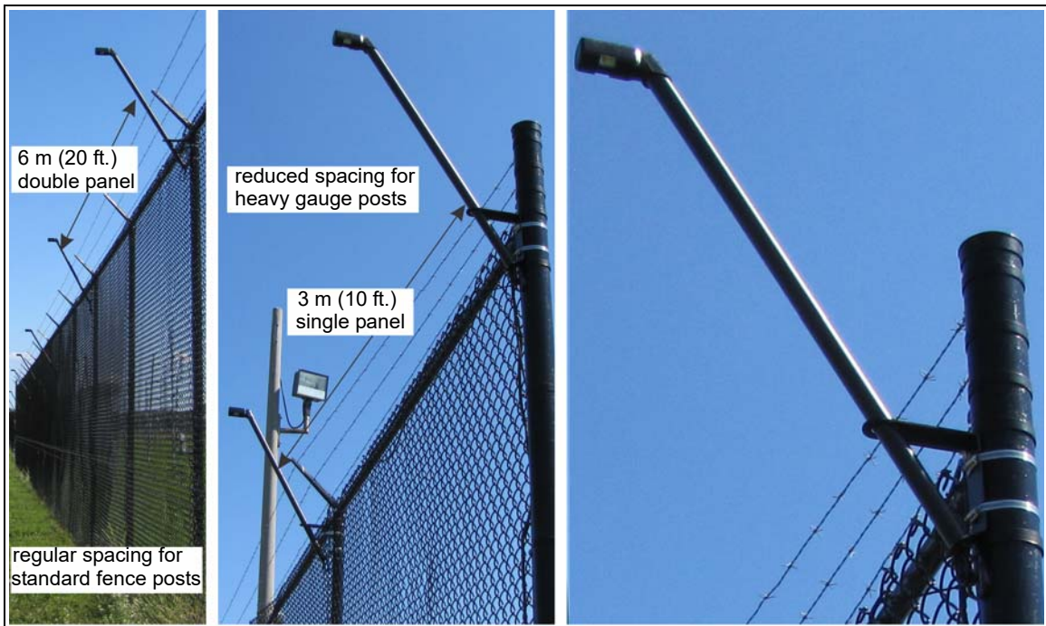
Figure 15: Luminaire installation on heavy gauge posts
