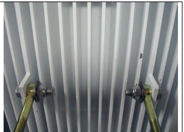
ODU top elevation rod attachments
