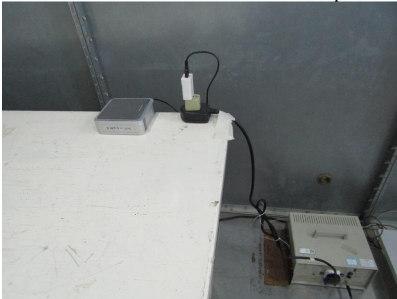
Measurement of Conducted Emission Test Set Up
