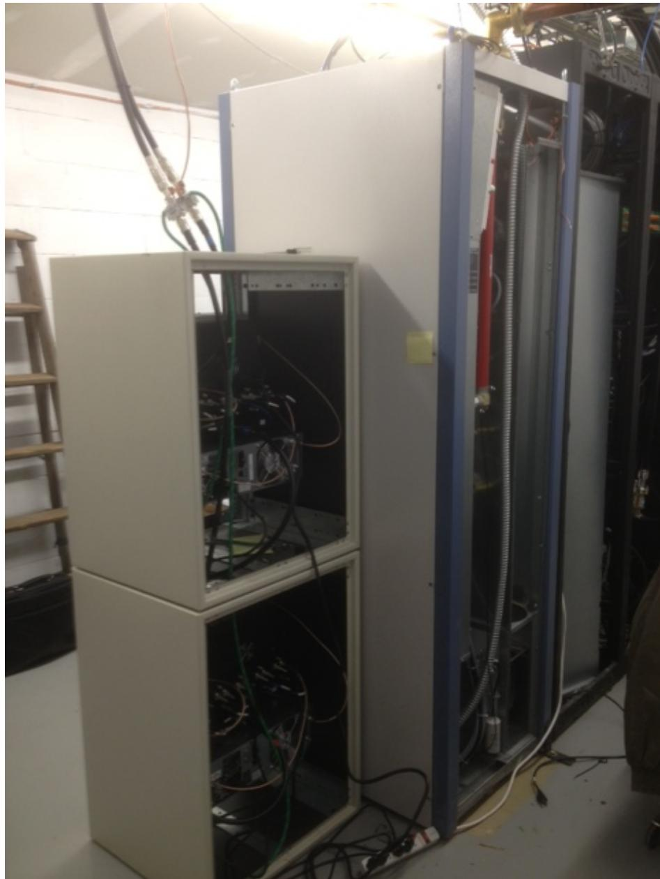
The transmitter is sandwiched between two other racks. This picture of the right side of this transmitter is taken from a different angle than the previous picture. The flat metal skin that runs the entire length down to the floor can be seen here. In this picture the back door has been removed and the yellow material on the side of the cabinet is a temporary Post-It Note.
