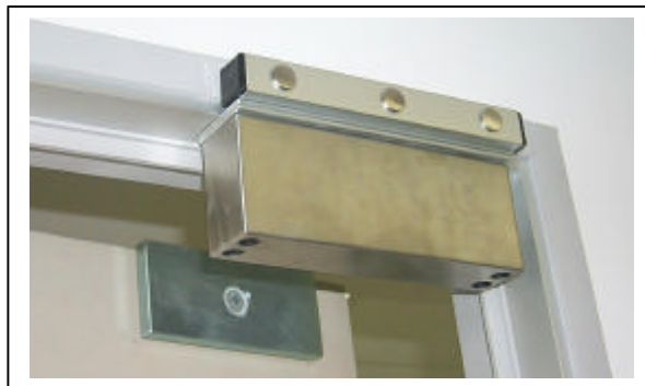
Figure 15 - Maglock Installation
