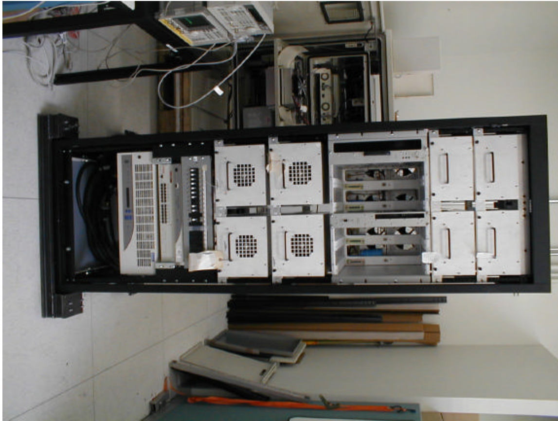
WCS RACK Top to bottom • 3 DARS Band reject filters • Power amplifier shelf, (1 PA installed, others removed to show detail inside the shelf, behind the PA's) • 4 WCS Radios • Power Supply circuit breakers • Ethernet Hub • -48VDC supply
