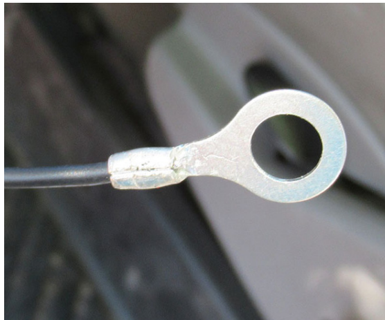
Figure 3 – Crimp Ring Terminal onto Black Wire
