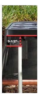
If you cannot drive the rod in enough to equal the necessary spacing, cut the remaining rod length to the proper height using an abrasive cut-off tool.
