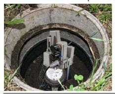
**Caution** Verify the pit lid does not touch the ERT module when the lid is replaced. There must be a 1 to 2-inch space between the top of the ERT module and the bottom of the pit lid. If the ERT module is installed too high, too low, or is touching any of the surrounding surfaces, adjust as necessary.
