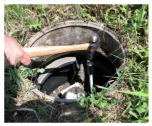
**Note** The rod shown has an end cap to protect the rod while driving it into the ground.
