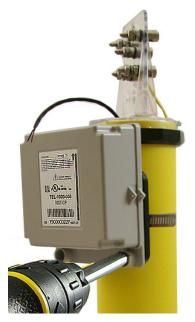
15. Install the tamper seals in the screw mounting cups. A tamper seal is correctly seated when it is recessed 1/16" into the cup.
