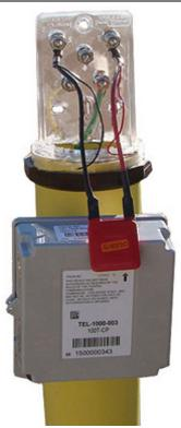
3. Connect the 100T-CP lead wires to the lightning suppressor following the table indications.
