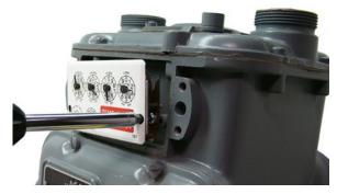
Set the index aside where it will not be damaged or fill with dirt, rain or snow. The index will be mounted to the endpoint later in this procedure. Verify the index mounting screws are 3/16" long and not corroded. If the screws are the correct length and not corroded, retain for later use. If the original screws were discarded, use the correct replacement screws (see Installation Prerequisites on page 7.)
