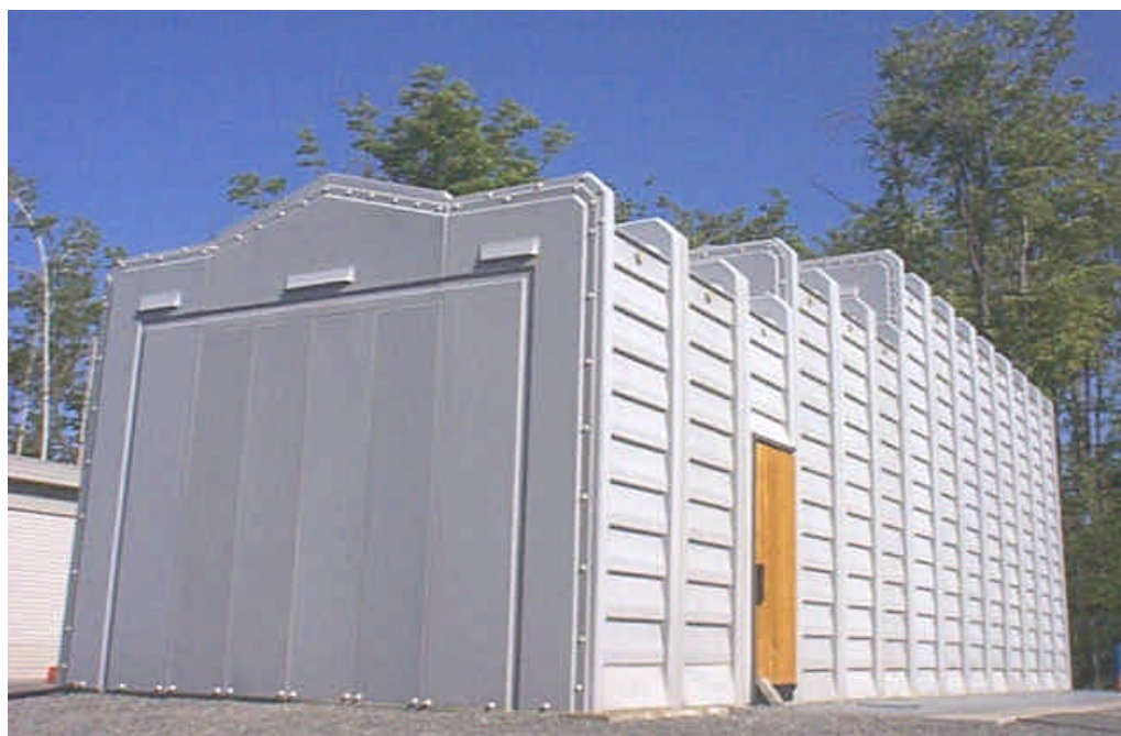
Fig. 1.b APREL's OATS (Open Area Test Site)
