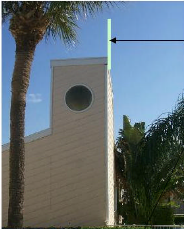
Figure 4 – Typical Mounting Location for the PET Repeater antenna
