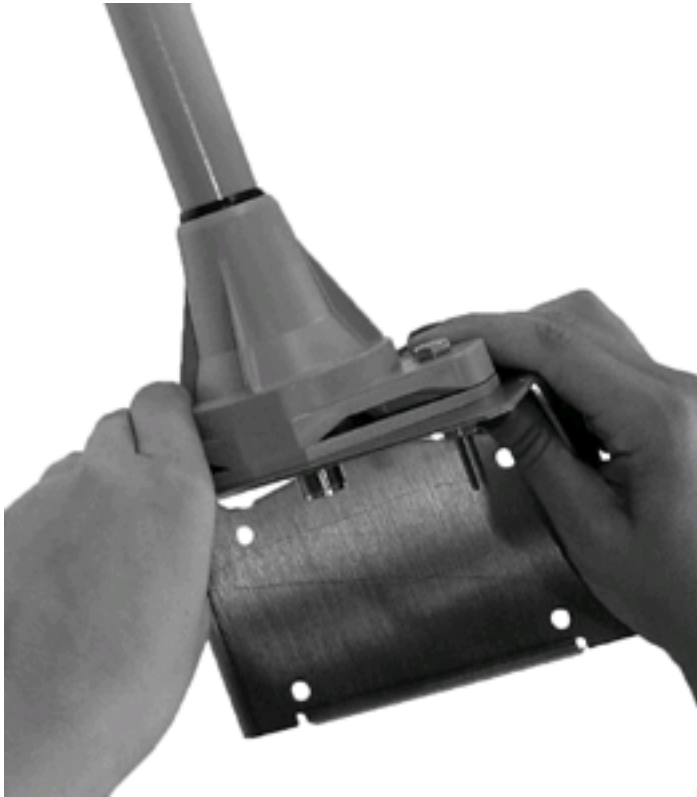
Figure 31 Remote antenna to IR8140 mounting bracket
