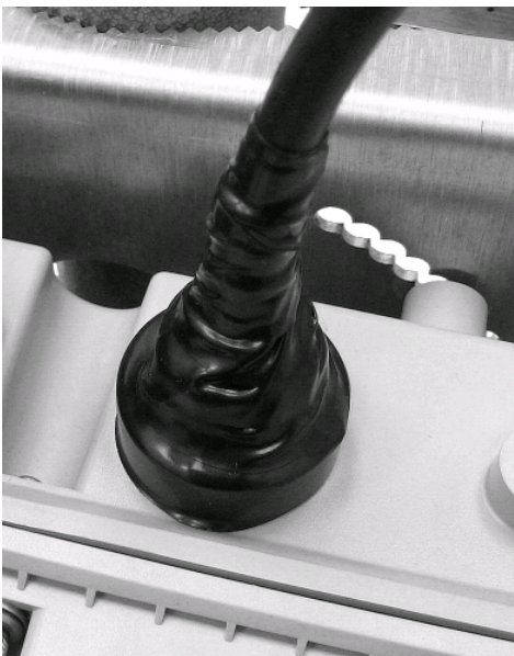
Figure 33 Fully covered electrical tape application
