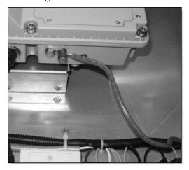
4. *(optional)* Connect the Ethernet cable to the CCU and the top of the 10/100 BT SPD. Feed the external Ethernet cable through the Roxtec block and connect it to the bottom of the 10/100 BT SPD.
