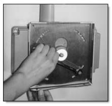
4. Using two steel straps, attach the mounting plate to the pole.
