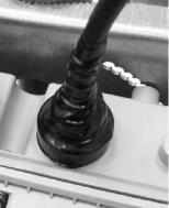
d. Wrap a layer of butyl rubber sealant over the vinyl electric tape.Ensure that the butyl rubber extends past the vinyl tape and onto the cable jacket.
