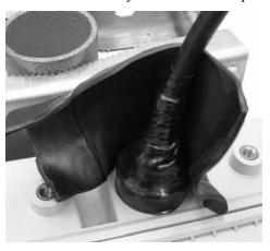
e. Overlap the butyl rubber so there is no gap. The butyl rubber will self-vulcanize over time and the seam will disappear.
