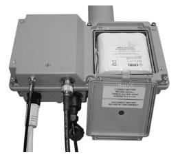
2. Plug in the four pin battery wiring harness. The harness should snap into place, providing a secure connection.
