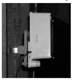
The adapter-plate mounting lug should be just above the ERT-module mounting lug recess.
