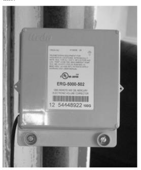
**5.** Tighten the screws to 9 to 12 inch-pounds of torque.
