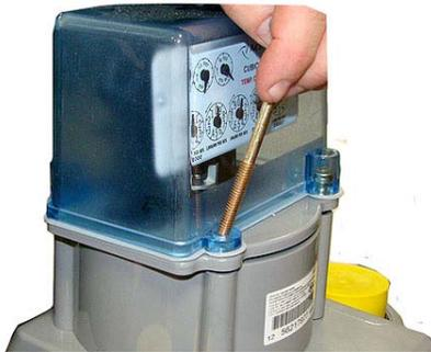
6. Insert tamper seals in the tamper seal cups on the index cover and press into place with an 11/32 nut driver or similar blunt tool.
