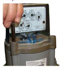
**6.** Place new tamper seals over screws (if mounting plate has tamper seal cups) and press into place with an 11/32" nut driver or similar blunt tool.
