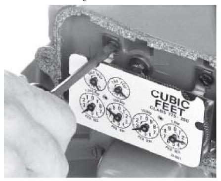
**5.** Remove all traces of the old index cover gasket from the meter. The new ERT module has its own gasket.
