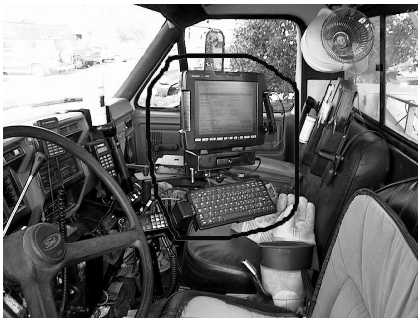
Photo 17: Shows another typical 6600 installation within a utility truck.
