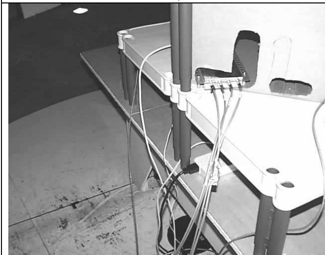
horizontal unit cable placement
