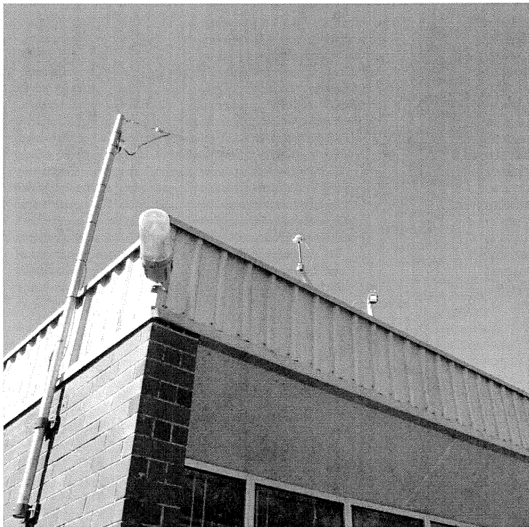
Photo of Semi-Delta fixed antenna ( Feed end )
