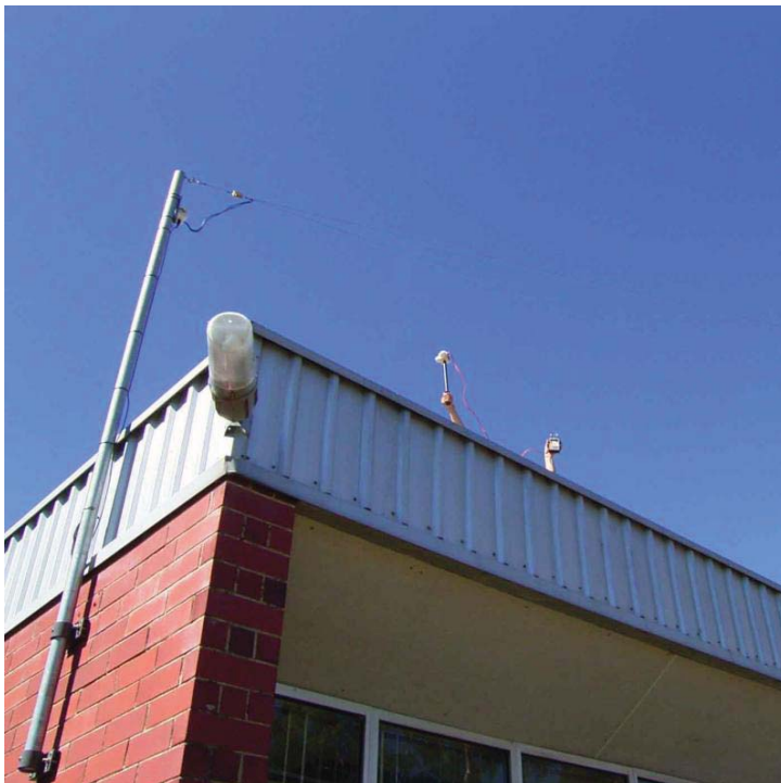
Photo of Semi-Delta fixed antenna ( Feed end )
