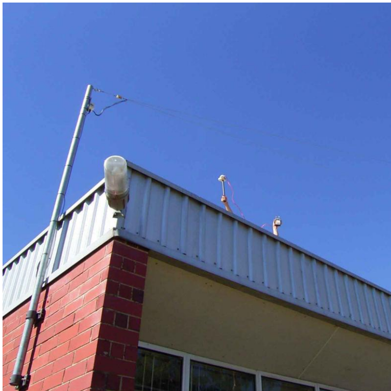
Photo of Semi-Delta fixed antenna ( Feed end )
