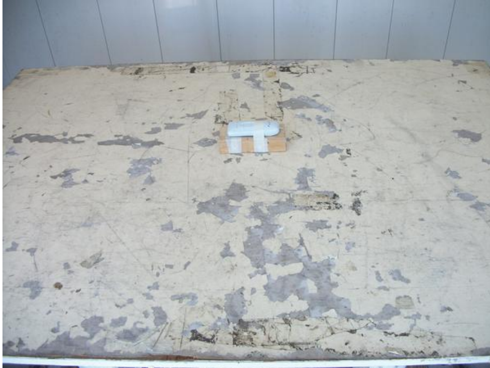
Figure 3.1 Radiated Test Setup, position 1-X
