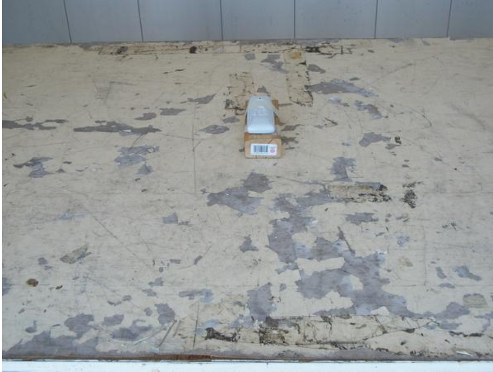
Figure 3.1 Radiated Test Setup, position 1-X
