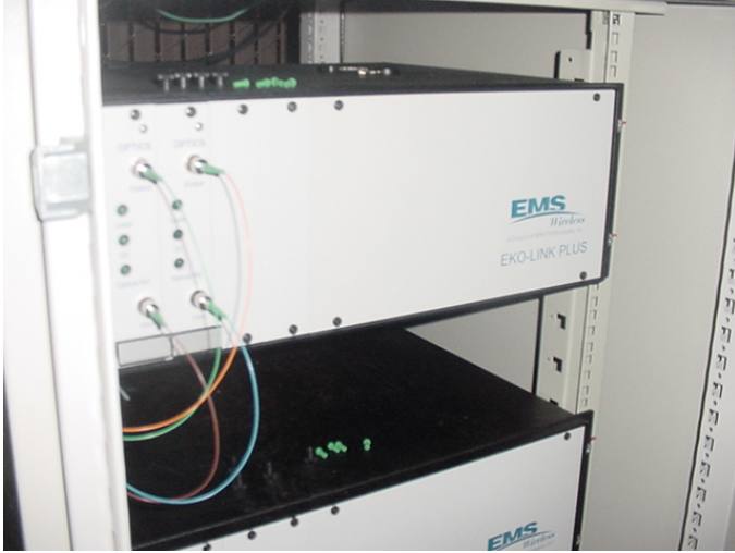
Figure 4: Rack Mounted EkoLink Plus Hub
