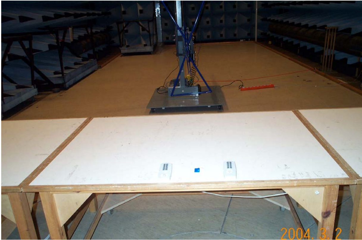
Photo 1 Set-up for measurements 30 - 1000 MHz. Date is correctly 2004-02-13.
