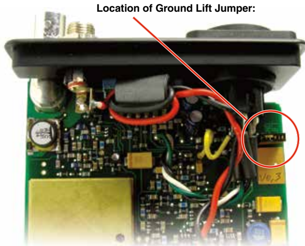
Jumper placed toward PCB as shown connects pin 1 to ground. Move jumper to outside contacts to lift ground.
