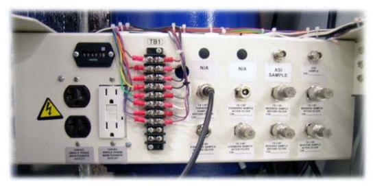
AC Distribution System Panel with AC Hour Meter and IF and RF Sample points
