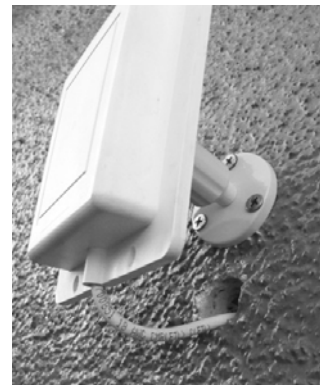
Figure 7. Antenna cable inserted through hole in wall
