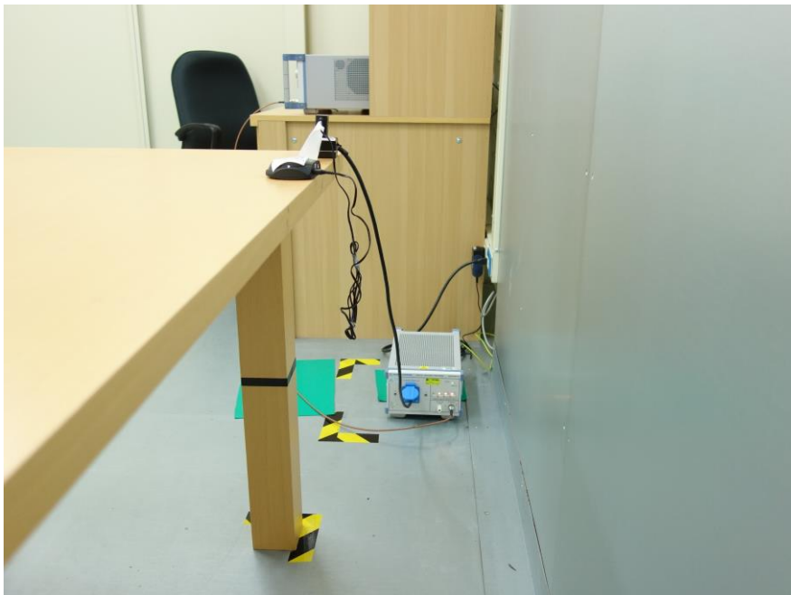
Photograph 8: Set-up for AC Mains (Back View)
