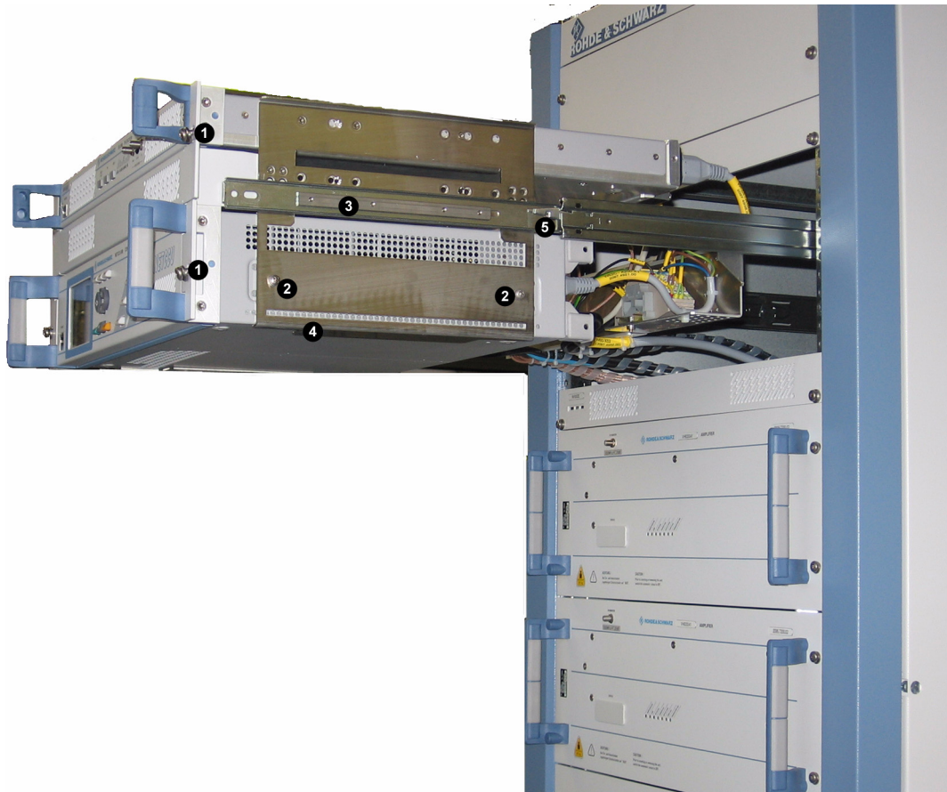
Fig. 12 Removing the NETCCU from the transmitter rack
