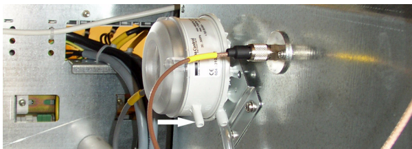
Fig. 7 Differential pressure gage without cover
