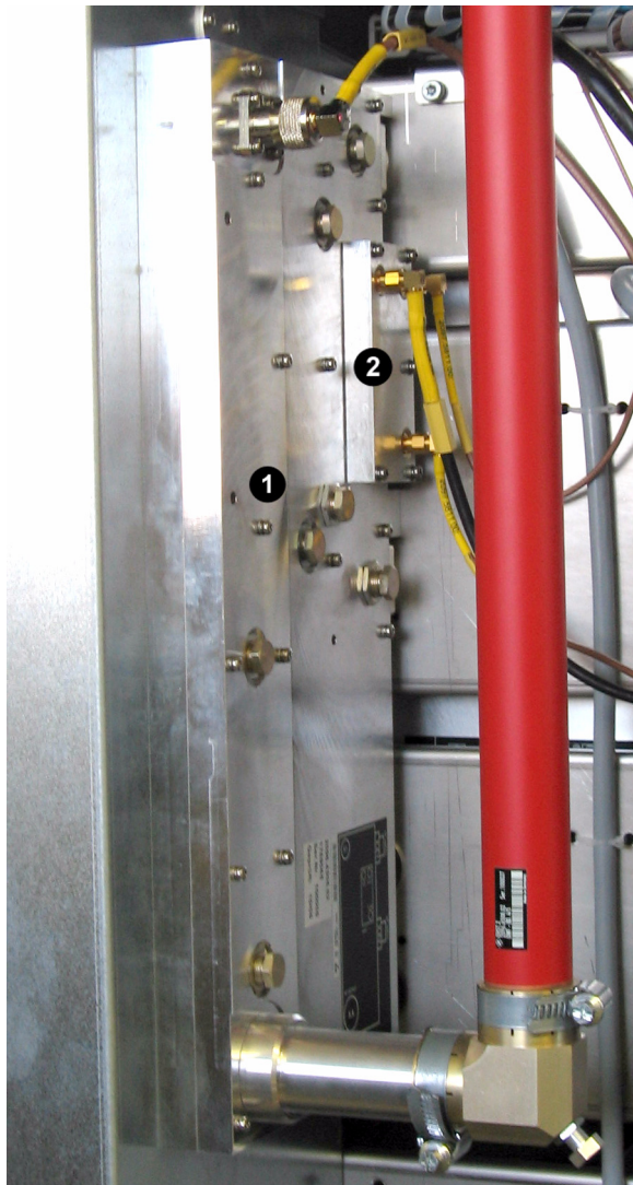
Fig. 23 Combiner (1) with splitter (2)
