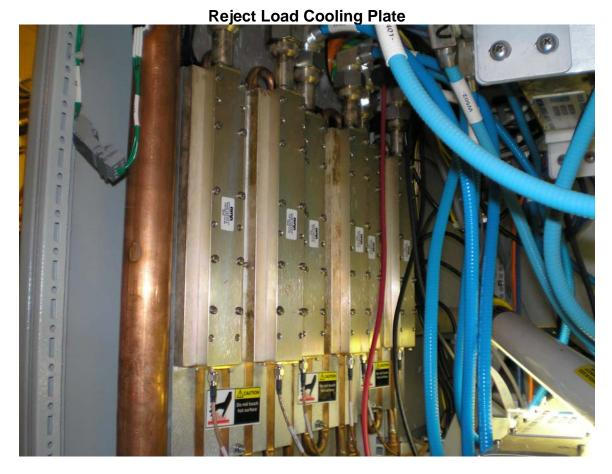
This photo is of the reject loads mounted on the cooling plate.
