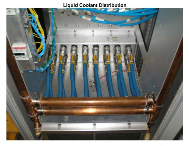
In this photo, the coolant distribution to the input and output connections of the either modules can be seen.
