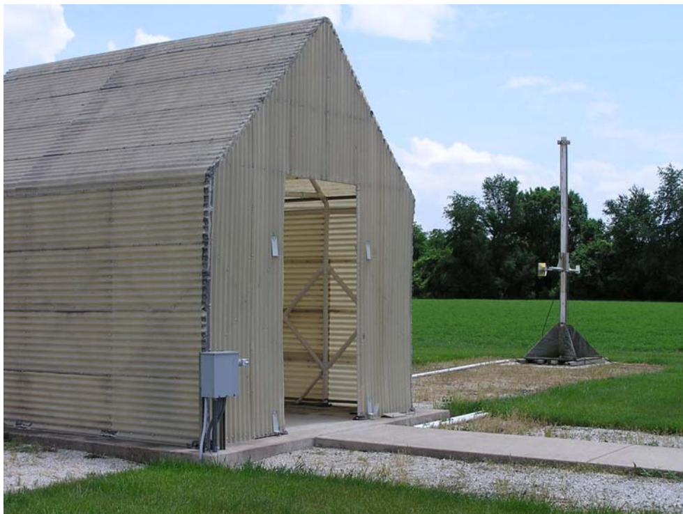
OATS Shelter Building, showing EMI Antenna Mast
