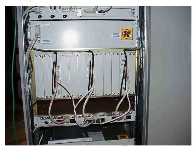
View: UMTS850 Macrocell Equipment Frame Front View Closeup, Showing the 25 MHz Dual Duplex Filter Shelf.
