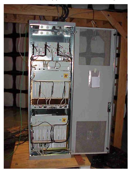
View: UMTS850 Macrocell Equipment Frame Front View Closeup, Showing the Digital Shelves with Multi-Carrier CDMA Radio (MCR850), BNJ65, and the Crystal Oscillator Module (OMA).
