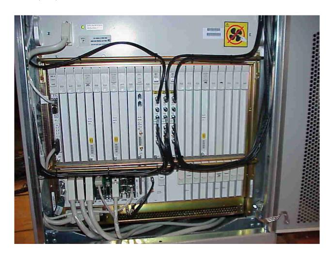
View: UMTS850 Macrocell Equipment Frame Front View Closeup, Showing the Power Amplifier Shelf.
