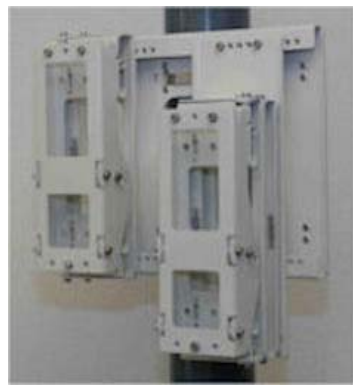
Tilt bracket assembly (double Metro Dock)
