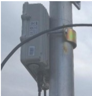
Figure 2-3: BreezeAIR basic mounting kit
