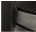
Figure 1b: Rack installation
