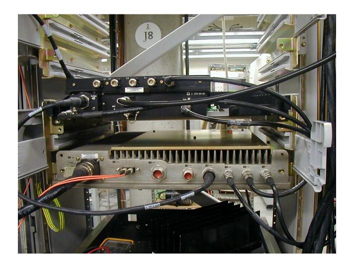
Nortel Networks MFRM2 Assembly Front View Fan Assembly Removed
