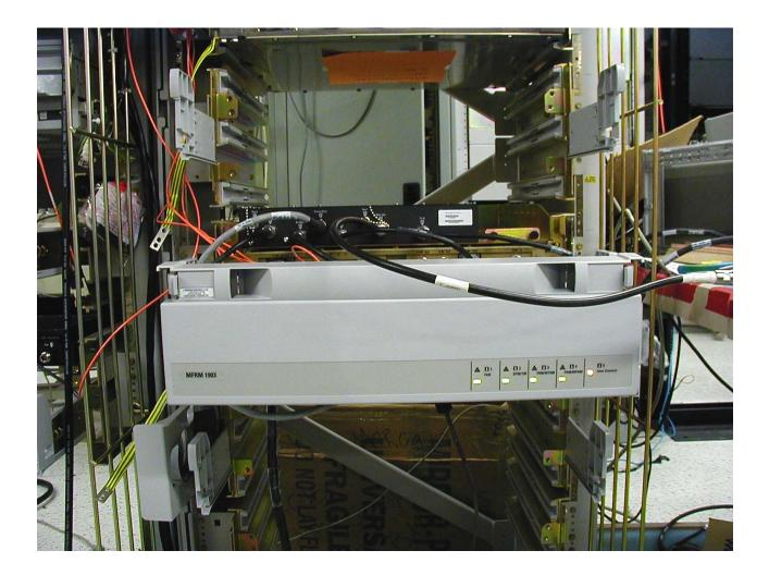
Nortel Networks MFRM Assembly Front View Fan Assembly Mounted
